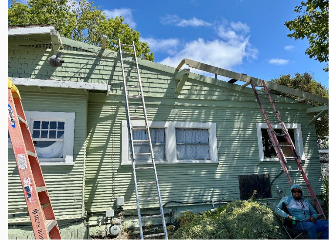
New roof for Annex
